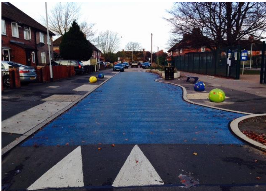
Figure 10: Traffic calming measures in Cannington Road
