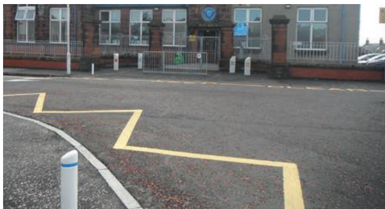
Figure 7: Raised junction outside of school
